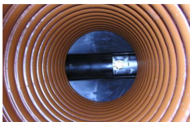
Photo 3. Push forward until the stopper on top of the Rat Blocker® is in contact with the pipe or the wall of the well. Turn the mounting pole clockwise until the Rat Blocker® is securely fastened against the pipe (it should not be over-tightened) and retract the mounting pole.
