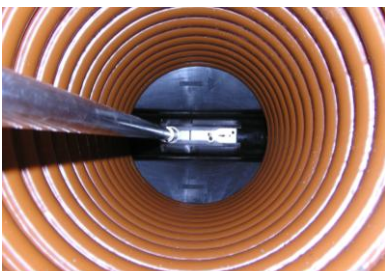
Photo 2. Lower the Rat Blocker and align with the sewer pipe. With gate in position 1, arrow must point against the flow direction; in position 2, arrow must point with the flow direction.
